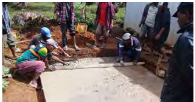
Anglicare PNG Volunteers creating the concrete slab box for the basement at Yaken Aid Post, Mendi SHP. (Photo credit: Anglicare PNG)
